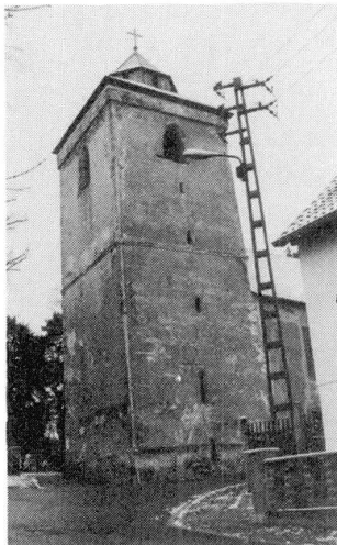
Fig. 1 : The bell tower, view from south-west
