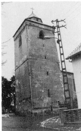
Fig. 1 : The bell tower, view from south-west
