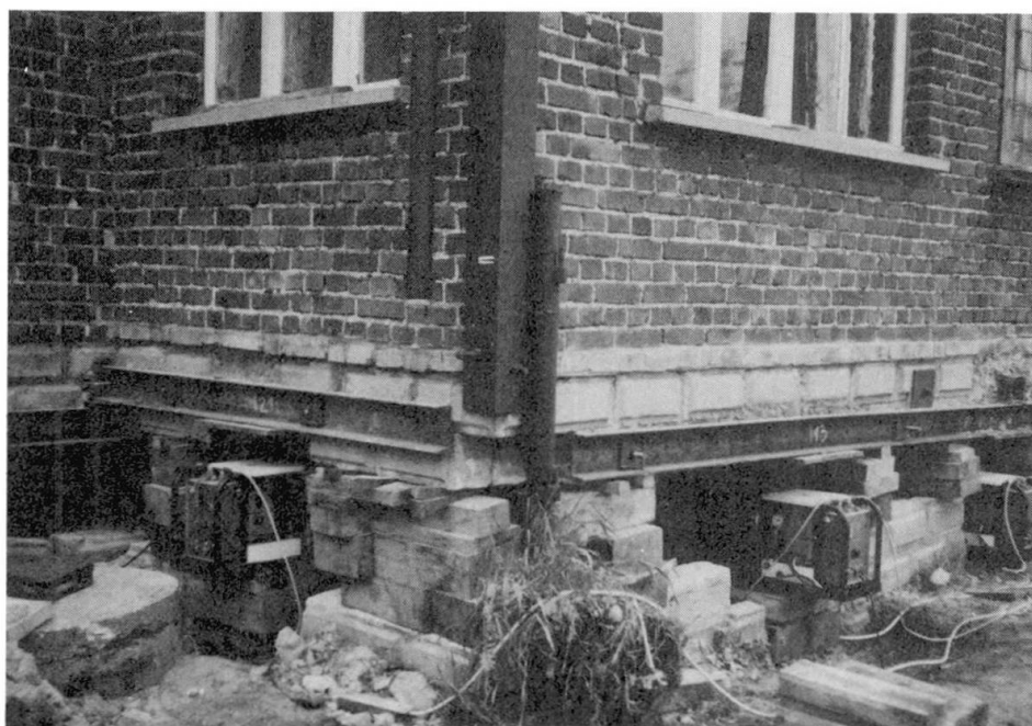
Fig.2 Built in jacks in cellar storey
