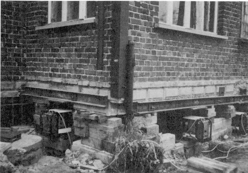
Fig.2 Built in jacks in cellar storey
