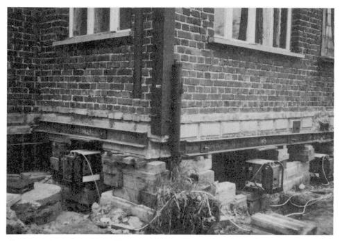
Fig. 2 Built in jacks in cellar storey
