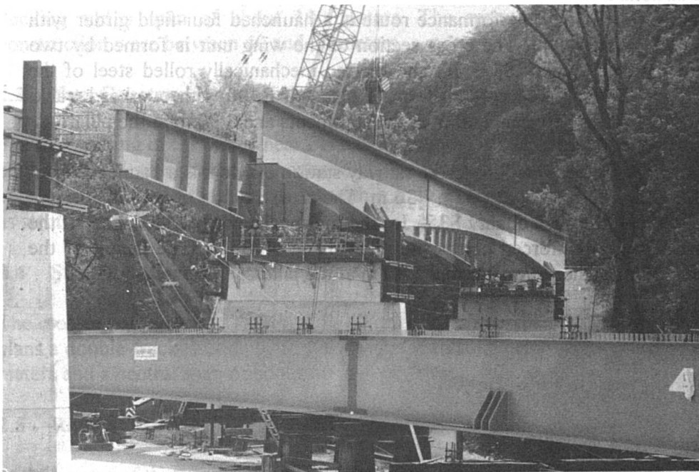
Fig. 2 Establishing and connecting the two main girders of the span crossing the river
