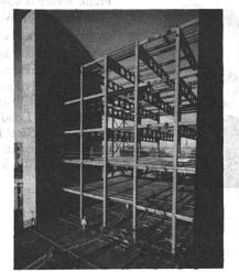
Long-Span Composite Cellular Beams
