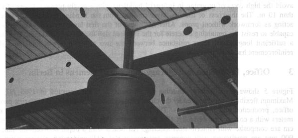
Fig. 6 Architectural shaped beam-column connection
