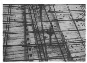
Fig. 4 Hilti connector. It consists of a glued threaded bar M12 which is post-tensioned after the setting of the concrete. The shear is transferred by grooves perpendicular to the span
