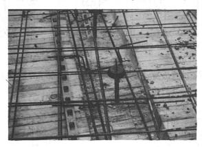
Fig. 4 Hilti connector. It consists of a glued threaded bar M12 which is post-tensioned after the setting of the concrete. The shear is transferred by grooves perpendicular to the span
