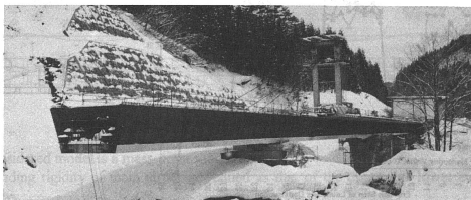
Photos-2 Incremental launching condition
