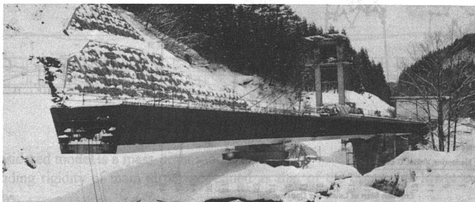
Photos-2 Incremental launching condition
