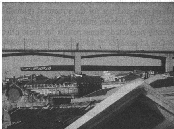
Fig.4 Launching phase of the viaduct
