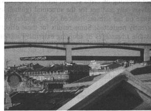
Fig.4 Launching phase of the viaduct
