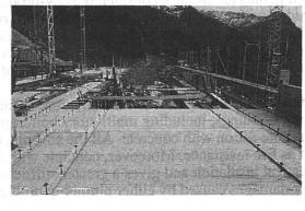
Fig. 8 - Wood elements and dowels for a timber-concrete composite slab: School in Triesenberg (FL).
