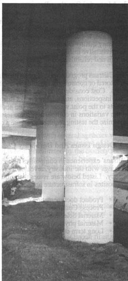
Figure 5 Application of Carbon Fiber ColumnWrap
