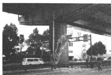
Fig. 1 Shear failure of a RC pier
