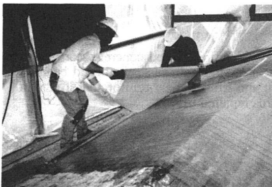
Fig. 1 Installation of Carbon Fiber Fabric
