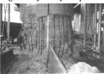
Fig. 2 Bending failure of a RC pier
