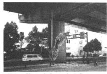
Fig. 1 Shear failure of a RC pier
