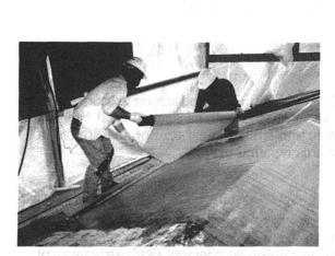
Fig. 1 Installation of Carbon Fiber Fabric &
