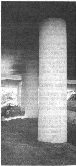
Figure 5 Application of Carbon Fiber ColumnWrap
