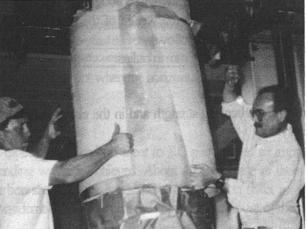
Fig.3. Installation of Prefabricated Composite Jackets
