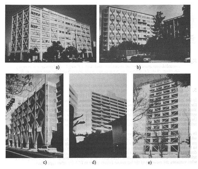
Fig. 11. Seismic upgrading of RC frames by means of steel bracings: a), b), c) Berkeley; Usual and Santa Monica - Los Angeles; e) Mexico City.
