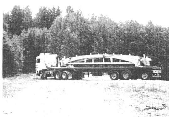
Fig. 5 Transportation of the edge girders to site
