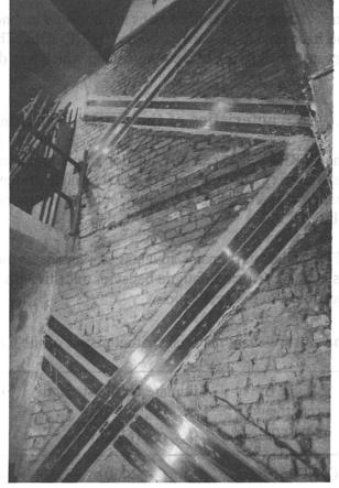
Figure 4: Distribution of CFRP-sheets on masonry
