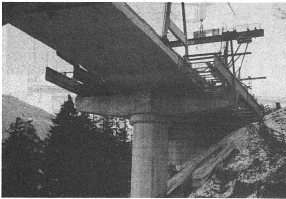
Fig. 7 Setting of steel units at outer structure
