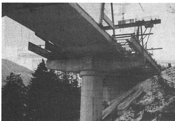
Fig. 7 Setting of steel units at outer structure
