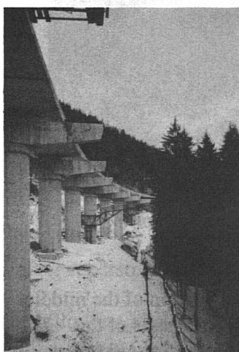
Fig. 4 Destruction outer deck slab
