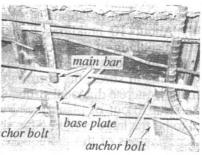
Photo. 3 Fracturing of Anchor Bolt at Column Base (after chipping concrete)
