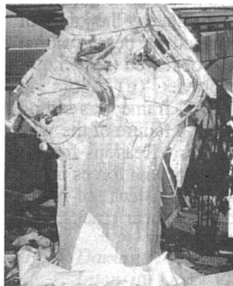
Photo. 2 Collapsed Column in Shear
