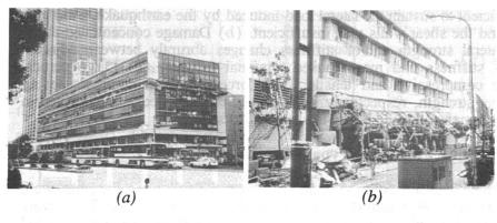
Photo. 1 Collapsed Building with Story Failure at an Upper Floor Level
