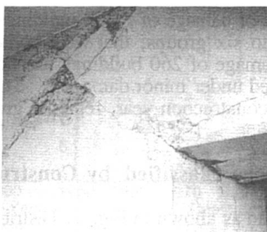
Photo. 6 Damage of Beam-Column Connection
