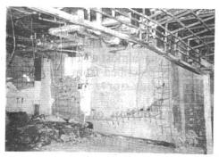
Photo. 7 Damage of RC Shear Wall
