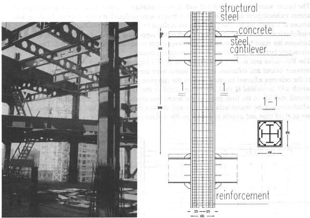
Fig. 5 Structural steel detail
