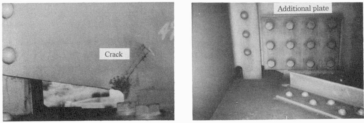
(a) Crack (b) Retrofitting method
