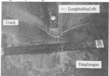
Fig.6 Damage of intermediate diaphragm
