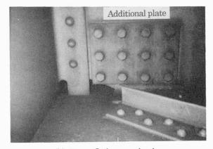
(a) Crack (b) Retrofitting method Fig.3 Damage and retrofitting of coped cross beam
