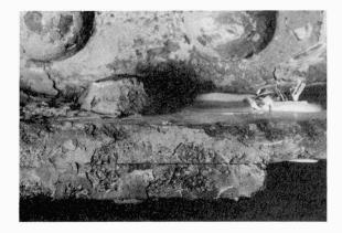
Fig. 6 Cracked angle in tension flange
