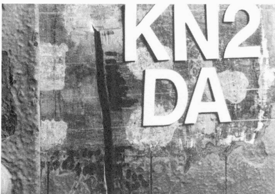
Fig. 4 Detail of crack tip in a web plate
