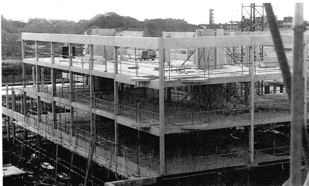
Fig.1. Typical precast concrete skeletal frame.
