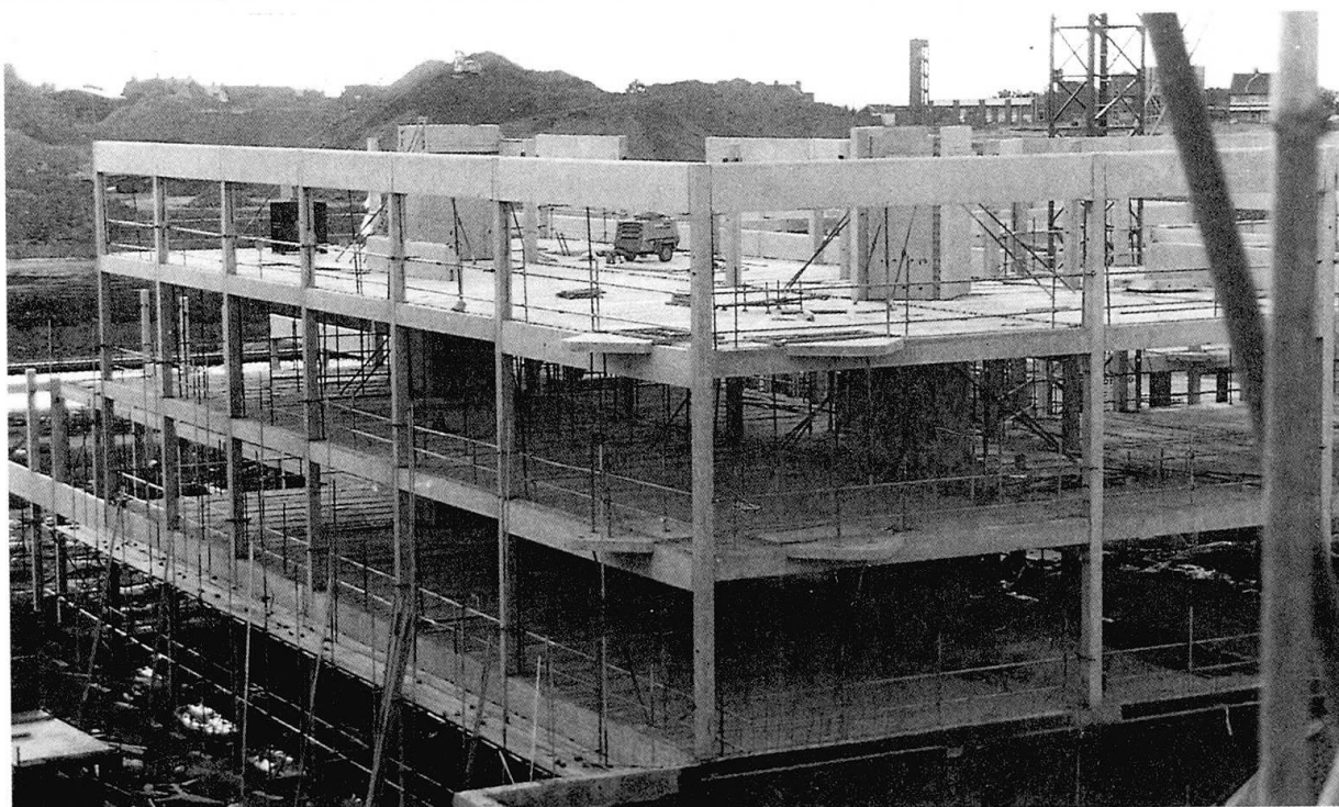
Fig.1. Typical precast concrete skeletal frame.
