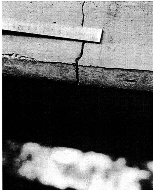
*Fig. 3. A Photo showing typical large cracks in RC beam of a bridge on TanZam highway.*
