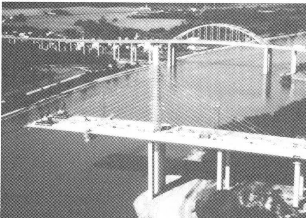
Figures 3.1 and 3.2 - Chesapeake & Delaware Canal Bridge, Delaware. Progressive cantilever construction of the 750' cable-stayed main span.
