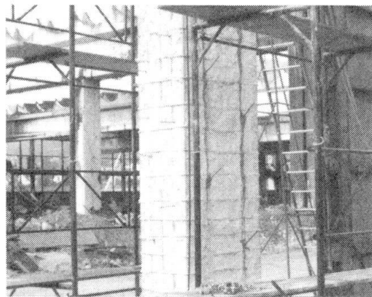
Fig. 4.2: A column core during the rehabilitation works
