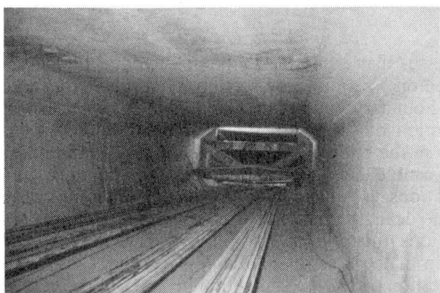
photo 13 - Prestressing cable system and deviation device frame
