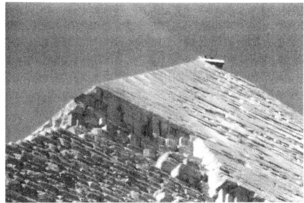
Fig. 2: Shifting of a block on the top of Chephren's Pyramid
