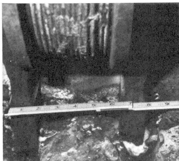
Figure 1. Corroded Eyebars on Manhattan Bridge
