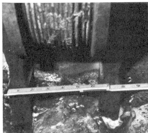
Figure 1. Corroded Eyebars on Manhattan Bridge
