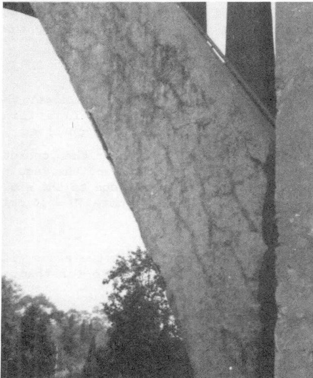
Fig. 2 Central Arch, southern view. Map cracking
