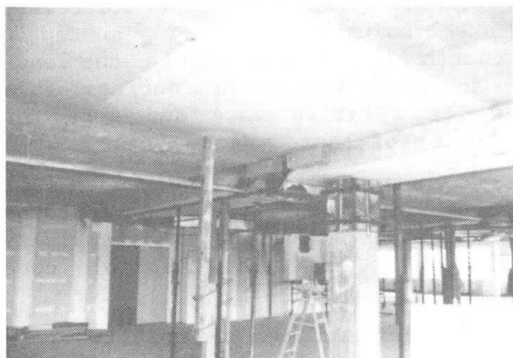
Fig. 3 External post-tensioning of transfer girders and steel collars confining column tops
