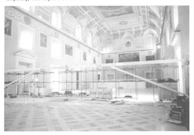
Fig. 4 Inside view of "Gran Salone" where a prosthesis prototype has been subjected to a load test.
