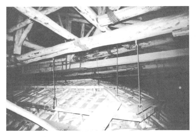
Fig. 2 Inner structure of wooden covering: lower trusses and depressed wooden vault with stiffening ribs before intervention.
