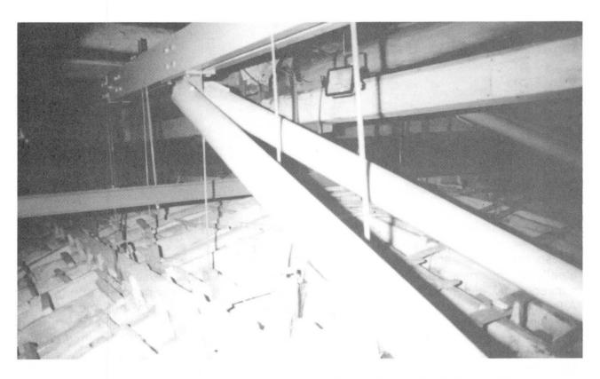
Fig. 6 New suspensions to steel prosthesis of the wooden vault after intervention.
