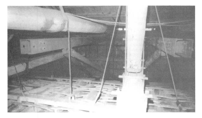
Fig. 5 Assemblage stages of prosthesis lateral beams.
