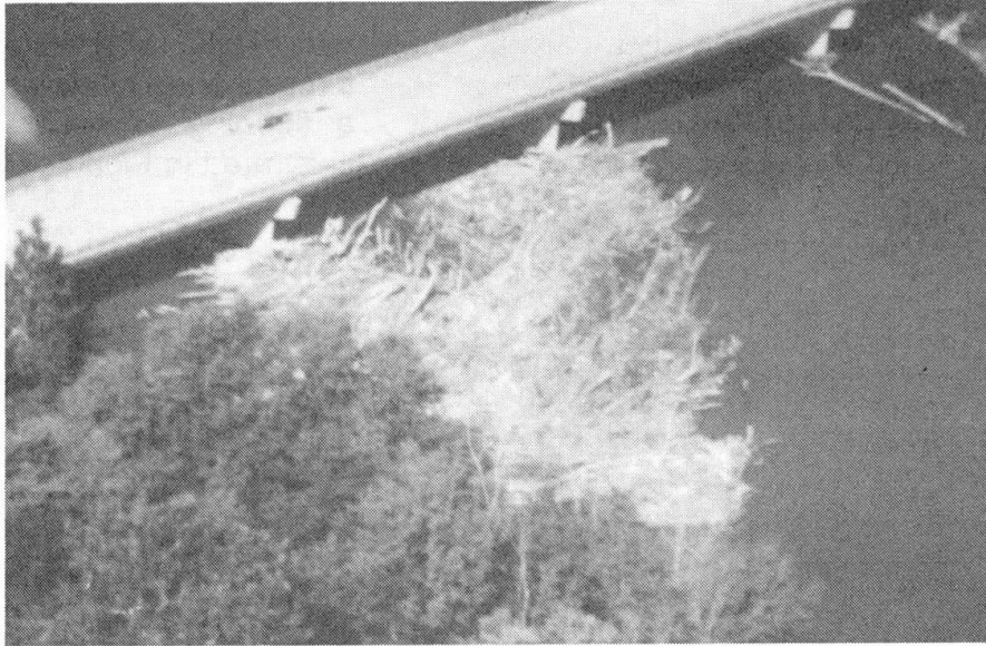
Figure 1. Typical Upstream Debris Accumulation
