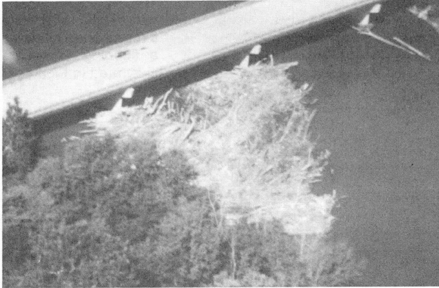
Figure 1. Typical Upstream Debris Accumulation
