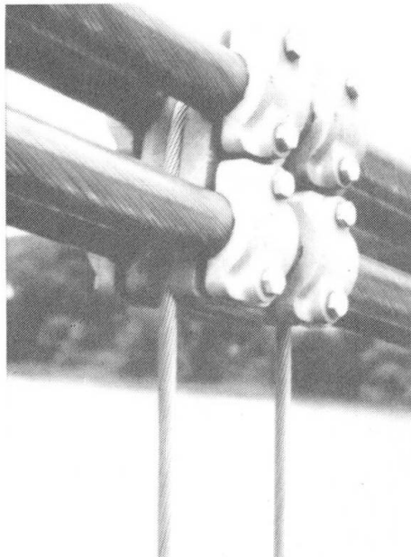
Fig. 7: Open rope bundles for large bridges. Gaps or slots must be avoided. Either care for close contact or provide ventilation and drainage.
