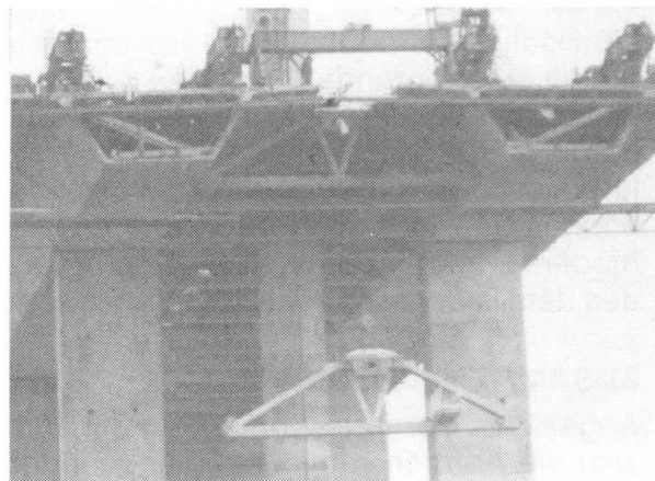
Figure 2.2 - Precast Delta Frames
