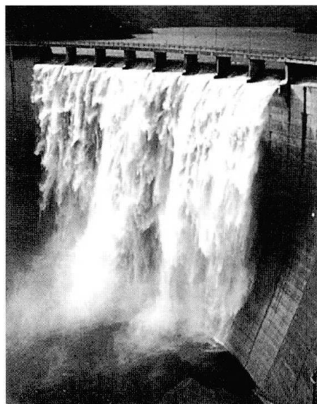
Fig.1 -View of the Ridracoli dam
