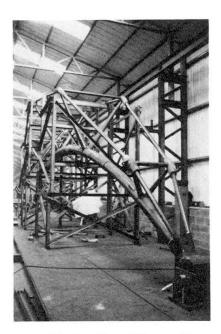
Photo 1. Minor Truss in the fabrication jig.
