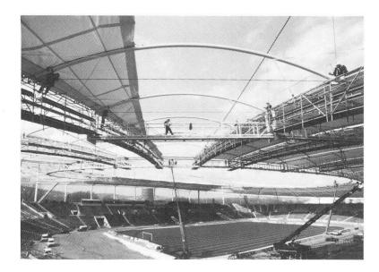
Fig. 16 Installation of membrane panels
