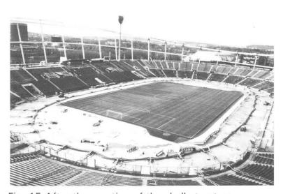
Fig. 15 After the erection of the shell structure the tension ring is assembled on ground
