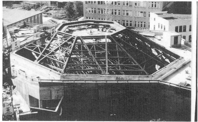
Fig. 3 General View of the Roof Construction
