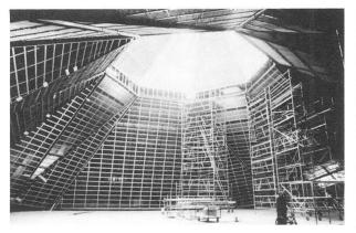
Fig. 5 Base Structure of the Hanging Ceiling
