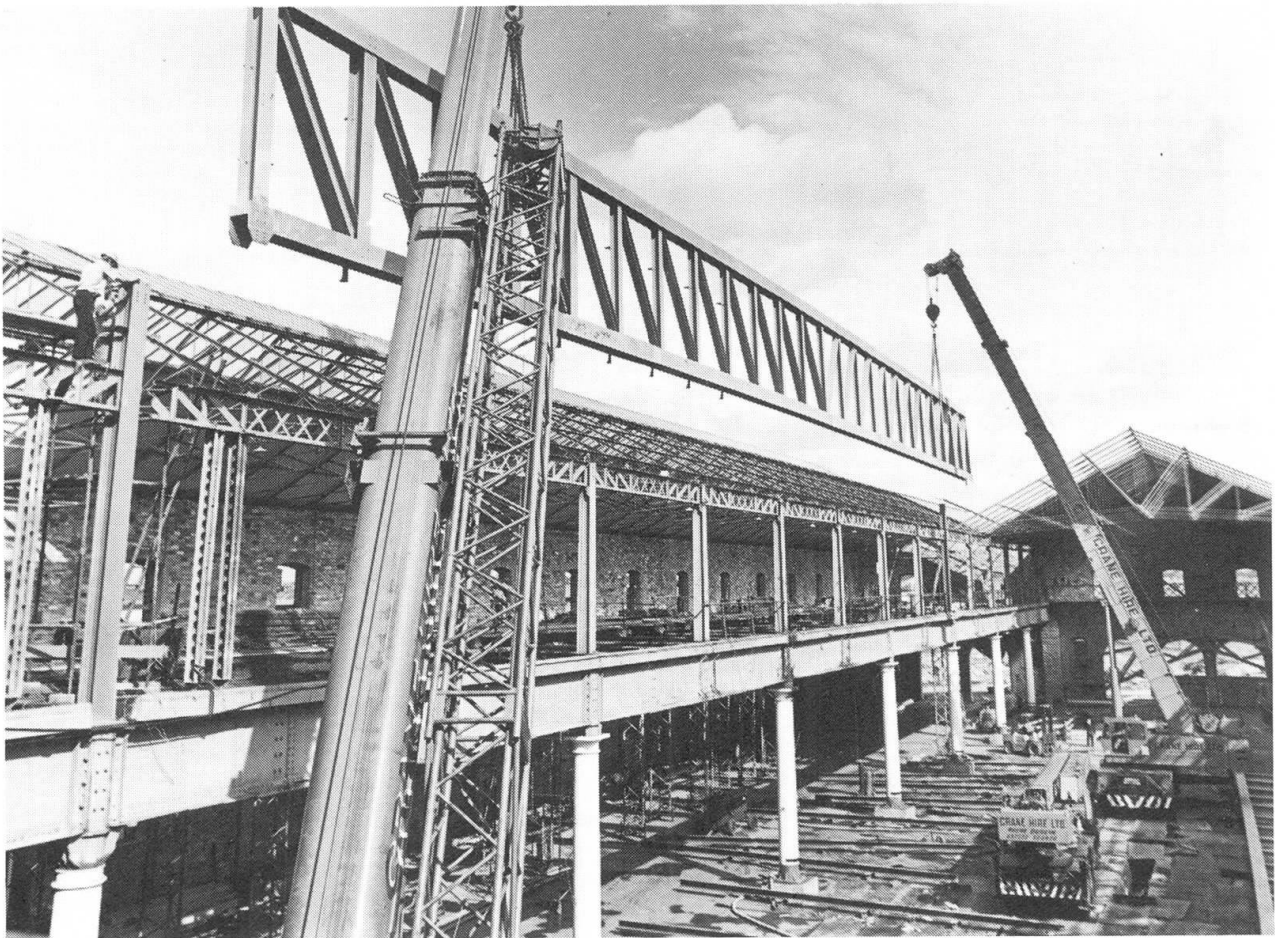
Fig.1: Erection of Main Roof Girders - Phase 1.
