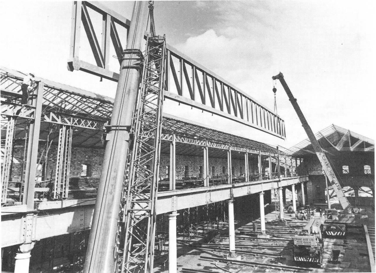
Fig.1: Erection of Main Roof Girders - Phase 1.
