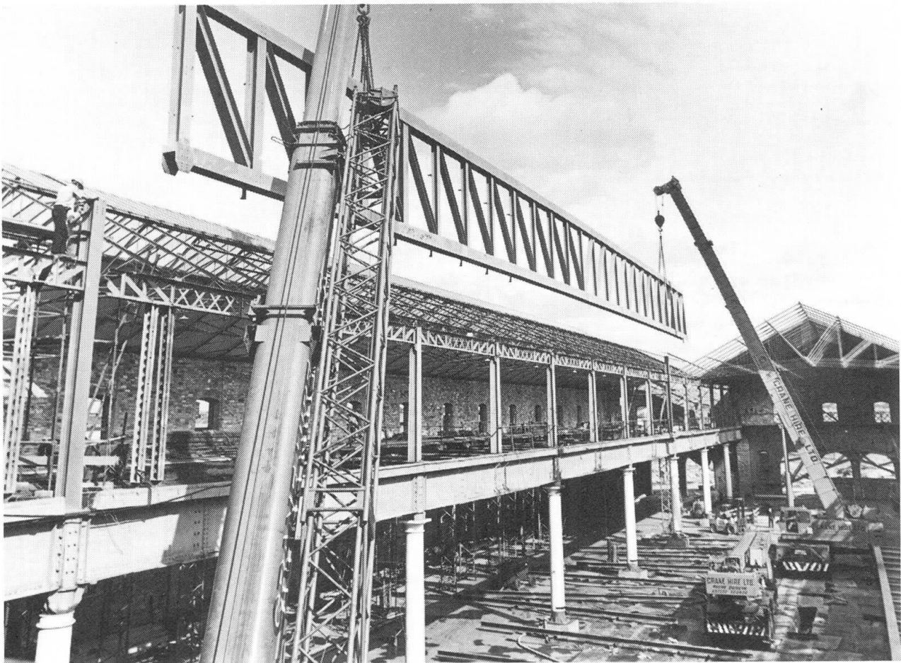
Fig.1: Erection of Main Roof Girders - Phase 1.
