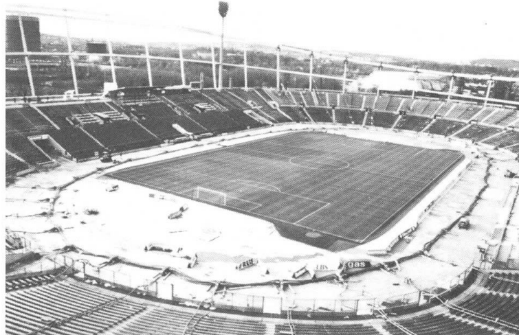
Fig. 15 After the erection of the shell structure the tension ring is assembled on ground
