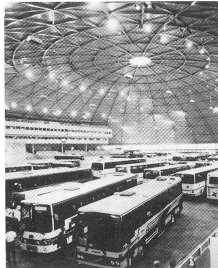
Figure 3 Inside view of the dome.
