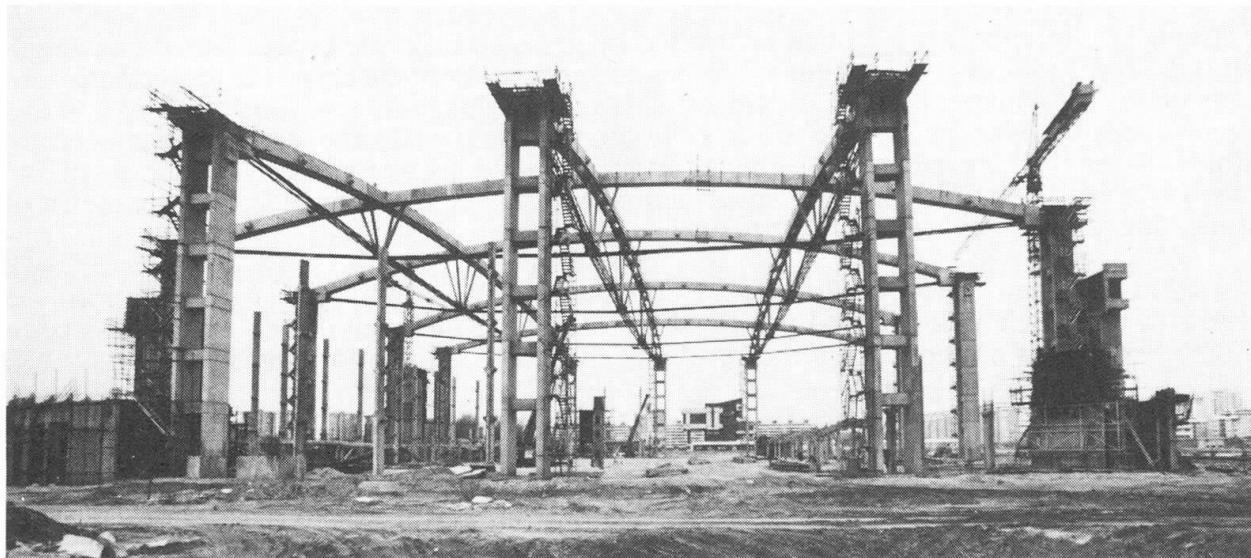
Fig. 5 Main roof girders in the final design position on the tops of the main columns
