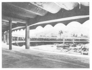
elements, each of 30 m span, 6.3 m wide and 60 t in weight. This element is cast on the ground in a timber mould and then erected / placed in position by means of a sophisticated erection scheme.
