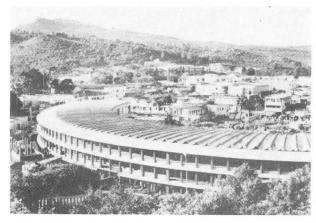
The pre-stressed channels are supported on brackets projecting from the RCC core walls, in a step-like fashion and form the upper gallery. The gallery steps are finished with marble. The lower gallery is formed by filling with earth and topping with PCC. Cut-outs in the core walls serve as passage for connecting the different compartments. (Fig. 7)
