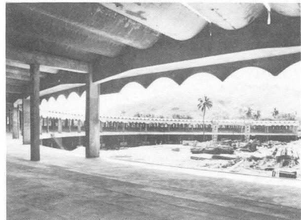
Prestressing was done by post-tensioning two cables, one of 21 m length comprising six 12.7 mm strands and another of 30 m length consisting of six strands using Gifford-Udall system. Each strand was given a force of 15T (Fig. 9)
